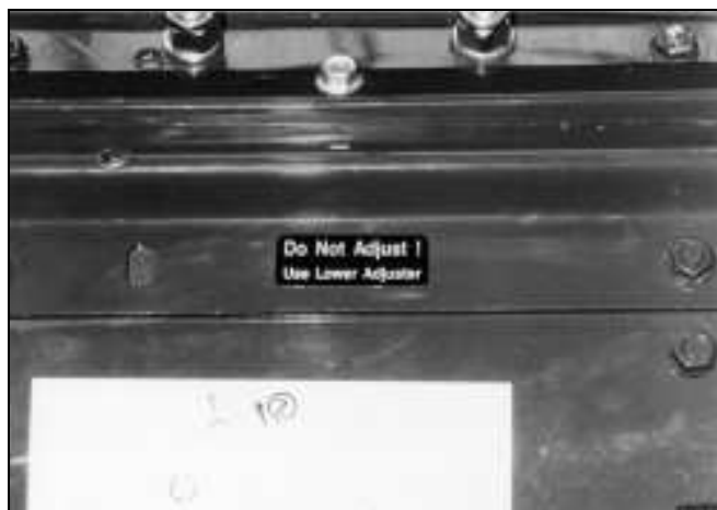
Figure 12. Decal installed on top of elevator
